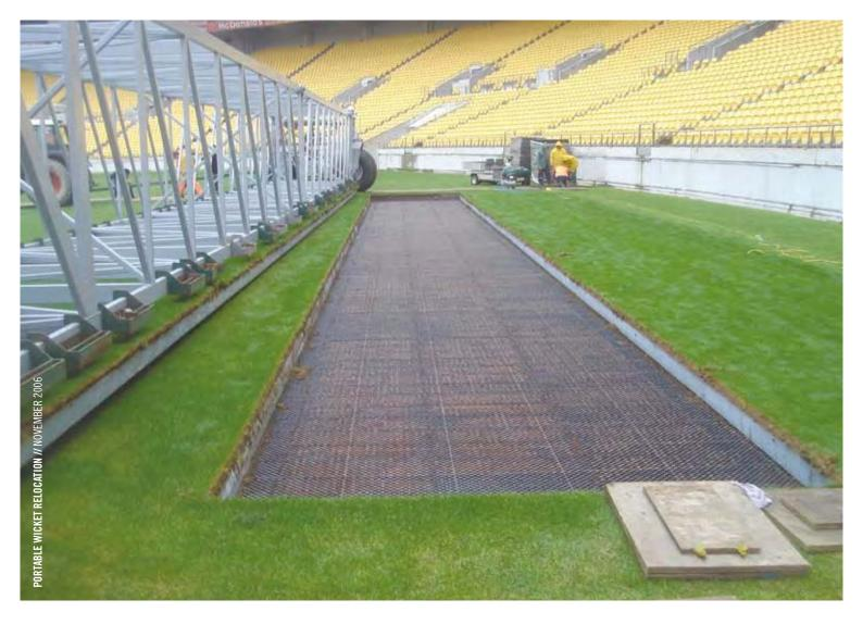
We own the steel frame, which is a major part of the specially designed transporter, and we hire the wheels and motor system from Eden Park when we need to shift the wicket, which is generally twice a year.
